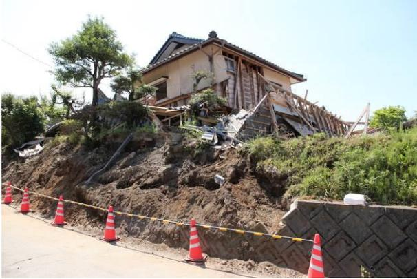
Figure 3. House damage due to collapse of retaining wall.
