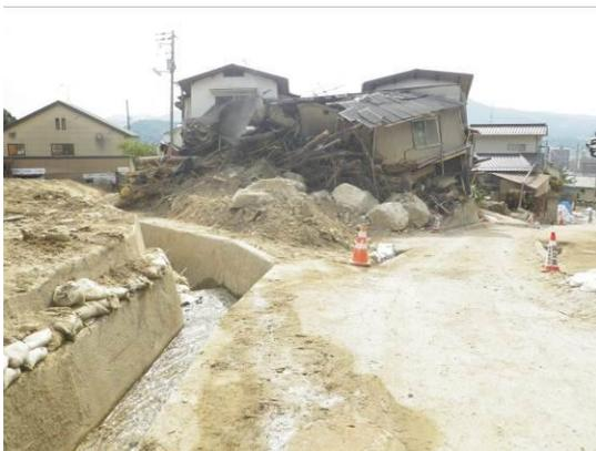
Figure 4. Debris-flow damage of houses in Hiroshima, 2014.
