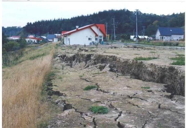
Figure 2. Damage of residential land resting on fill underlain by soft peat.
